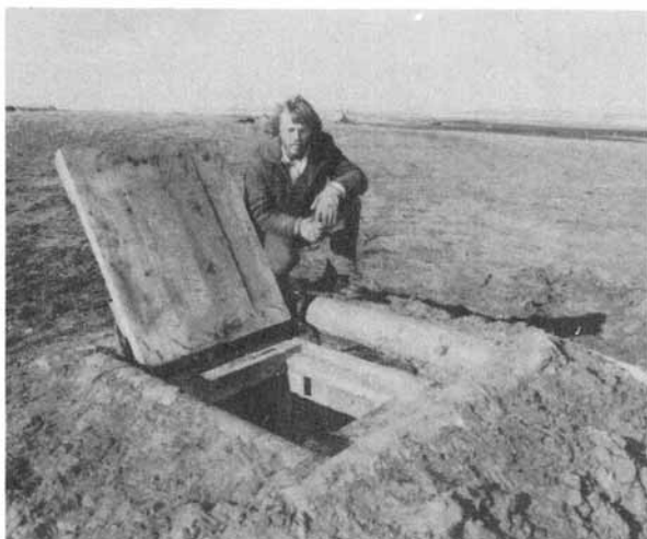
Fig. D.13. Blast door surrounded by 4 blast-protector logs that were notched and nailed together. The wet, mounded soil had been compacted by the blast but not blown away.
